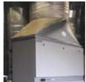
Example of duct installation
